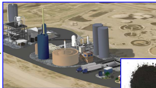
The Rialto Facility
